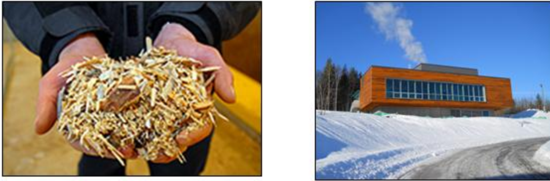
Figure 11. Wood waste used as fuel (left) for the bio-energy plant at UNBC (right), which extracts clean-burning gas from a local sawmill's wood waste to supply 85% of campus heating. (source: UNBC 2011)
