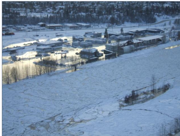
Figure 4. Recent flooding events in Prince George, such as the ice jam flood on the Nechako River in 2008, have affected road and trail transportation infrastructure.
