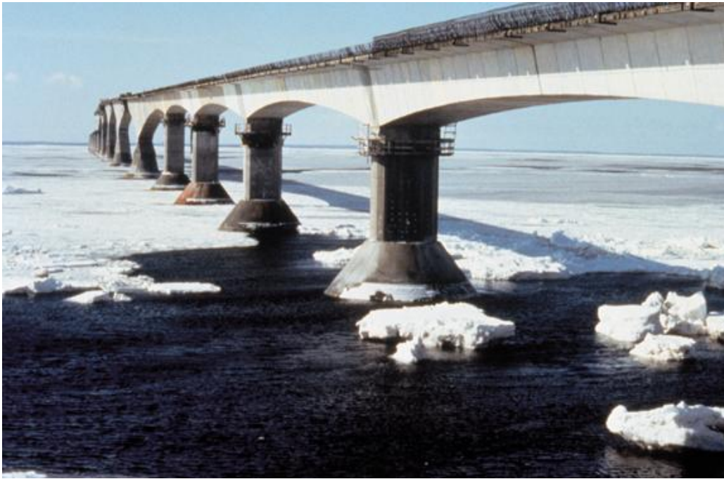
Figure 5. Confederation Bridge, which links Prince Edward Island to the mainland, was designed to account for 1 m of sea level rise. (Photo: from: www.concretethinker.com )
