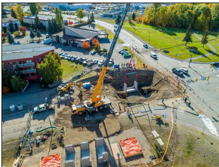
Figure 4: 2018 Winnipeg Street Storm Sewer Repair
