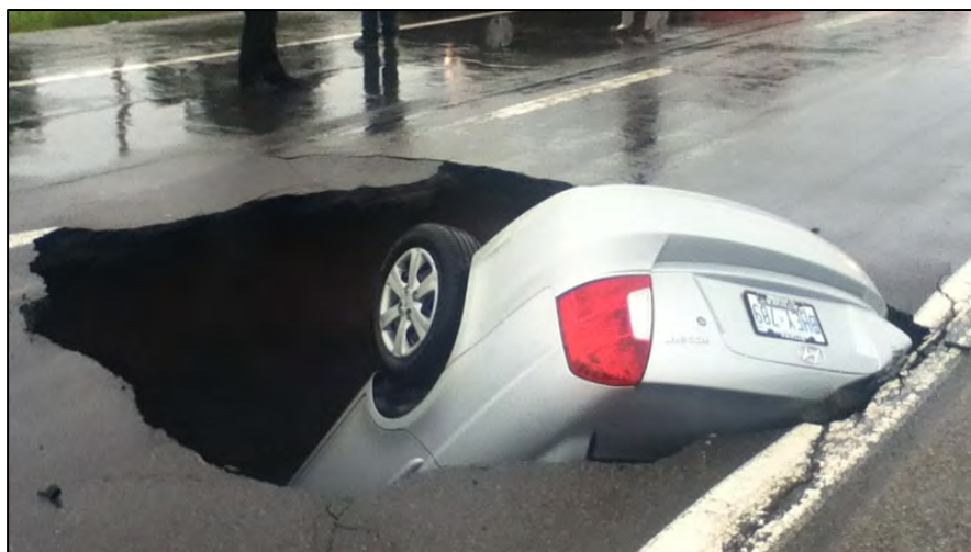
Figure 5: 2012 Sinkhole In Ottawa
