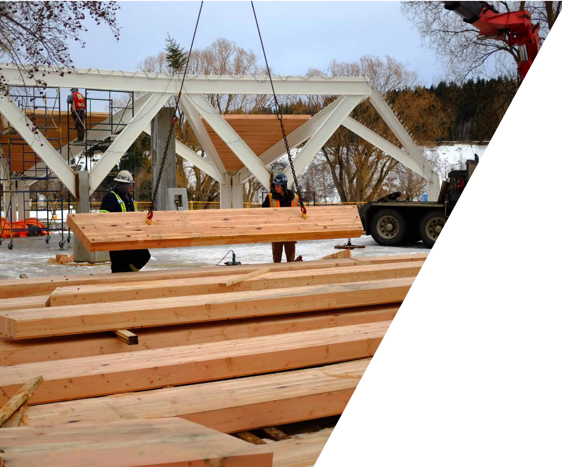
Construction of the Lheidli T'enneh Memorial Park Pavilion
