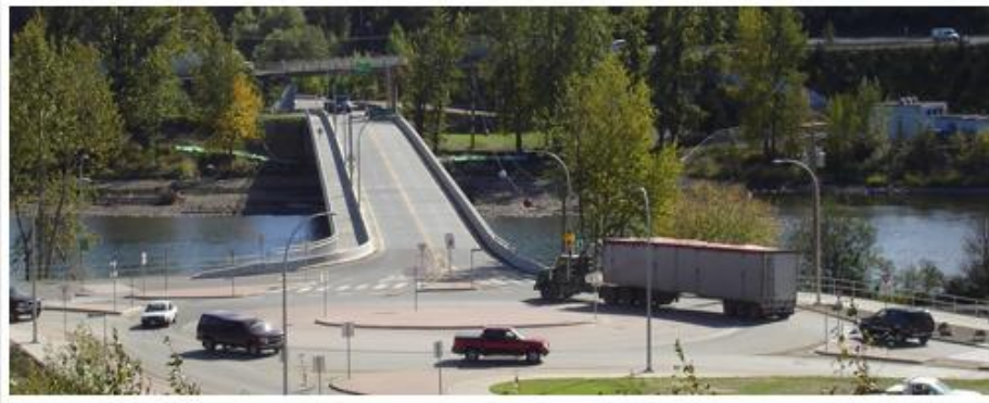
Current Cameron Street Bridge. Photo taken from north bank, circa 2010. Photo: City of Prince George
