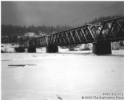
"Old Cameron Street Bridge." Photo taken from southwest bank, 1959. Photo: The Exploration Place, P991.9.2.17.1
