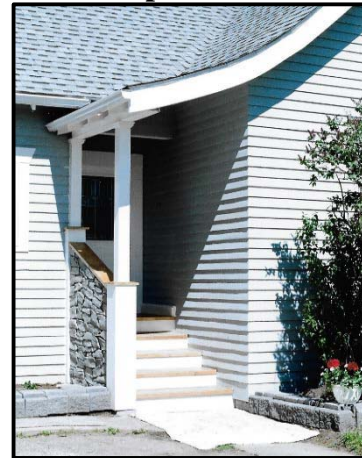
Bell-shaped roof at Entry
