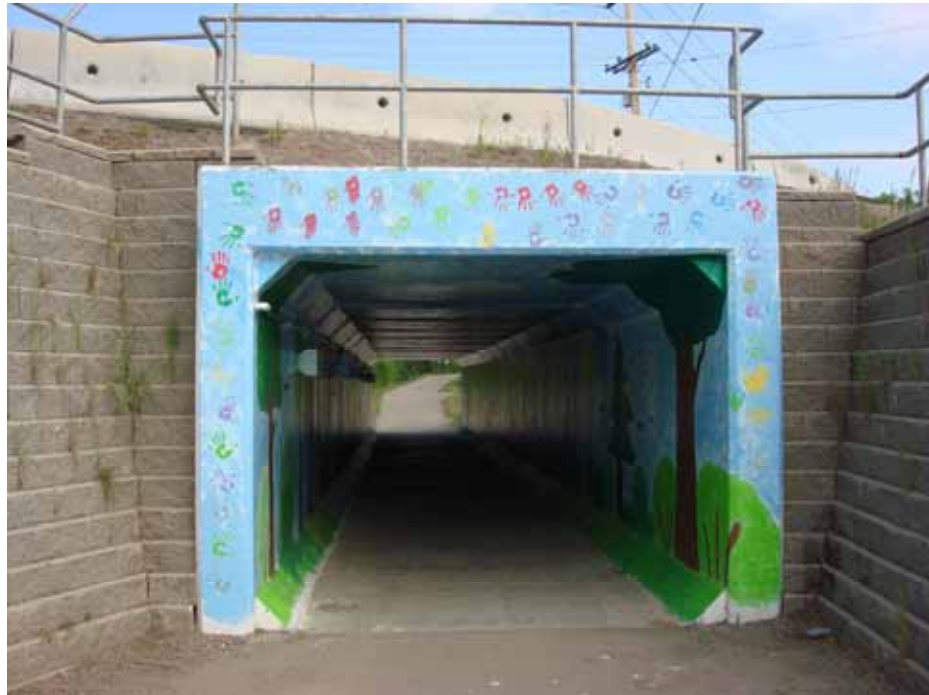
Figure 48 - Highway 16 Underpass at Heritage Trail
