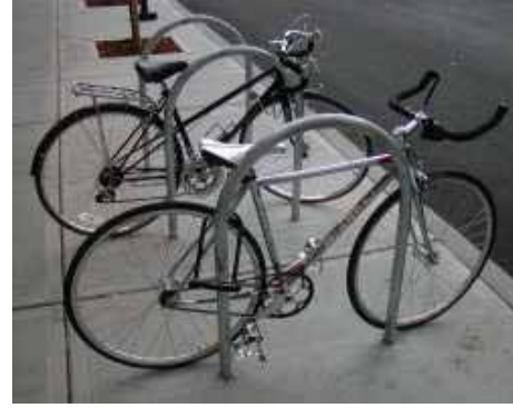
Frame-Supported: recommended
