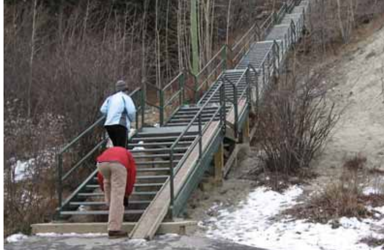
Figure 49 - Bike Rail on a Staircase
