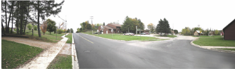
Intersection At Bobcaygeon Rd. and Parkside St. BEFORE
