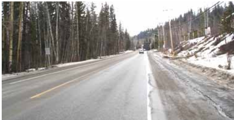
Figure 36 - Paved Shoulder, North Nechako Road
