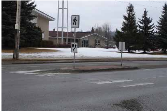
Figure 46 - Pedestrian Refuge Island, 5th Avenue at Voyageur
