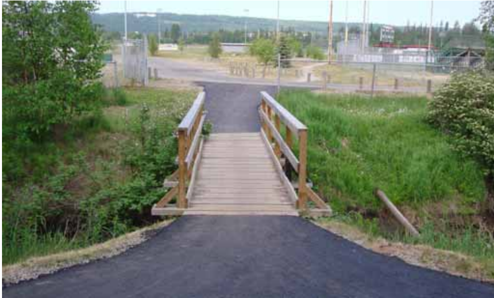
Figure 54 - Pathway Bridge in Carrie Jane Gray
