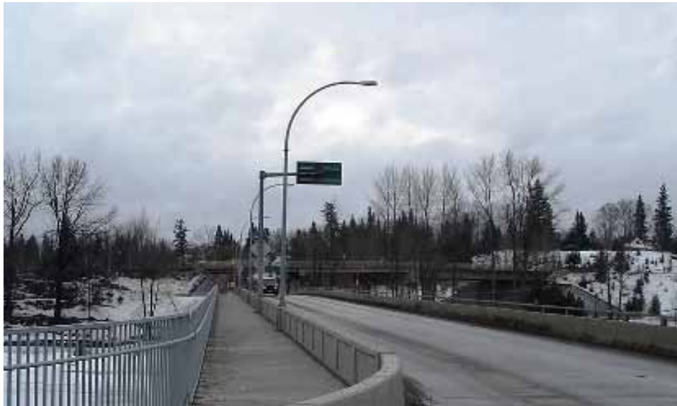
Figure 53 - Multi-Use Trail on Cameron Bridge
