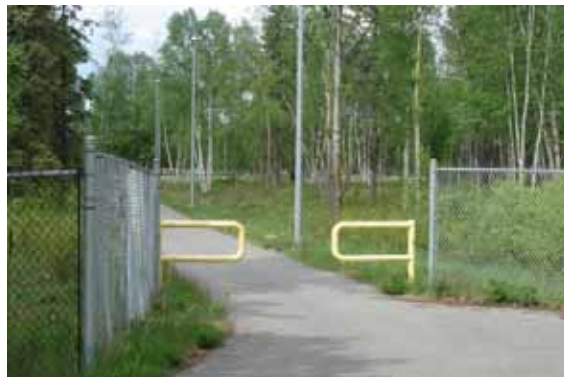
Figure 22 - Vehicle Barrier at the North end of the Cemetery Trail
