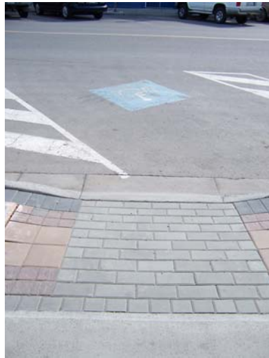
FIGURE 8.2 ACCESSIBLE PARKING STALL IN PRINCE GEORGE
